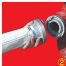
② 水带一头接在消火栓接口上 Connect one side of water pipe to fire-fighting hydrant
