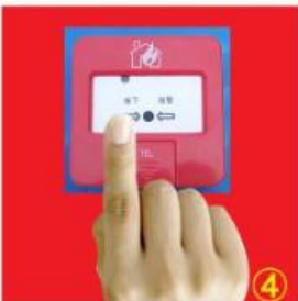
④ 按下箱内消火栓启泵按钮 Press the "start" button of fire-fighting hydrant
