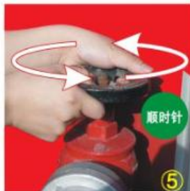
⑤ 打开消火栓上的水阀开关 Open the valve of fire-fighting hydrant
